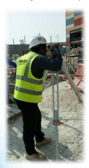
A setting out survey involves the marking out of any physical feature that appears on an engineering plan, in its correct position on the ground. These surveys are normally required during the construction of pools.
