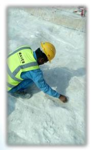
Blinding concrete to the required thickness as approved will be laid on a layer of 1000g polythene sheet over the prepared surface. The blinding concrete will extend a minimum of 200mm beyond the edge of the base slab. This is for the installation of sacrificial block work.
