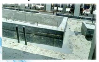
After curing of the concrete, cleaning and clearing the surrounds will start. All contaminated and waste materials will be removed and disposed of-site. Before back- filling commences, the subgrade will be watered, levelled and compacted.
