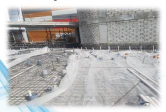
After the completion of the compaction and testing of the final layer, trenches for laying all the UPVC pipework below the base slab will be excavated and formwork in sacrificial block work constructed for the sumps. All pipework will be laid as per approved drawings and supplier's specifications, pressure tested for a minimum period of 24 hours prior to backfilling and levelling to the required profile.
