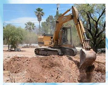
The area to be excavated shall be properly marked and clear before starting the works. As soon as the excavation reaches the required depth/elevation the surface shall be levelled and shall be compacted to required density. Before the compaction starts, it shall make sure that the excavated level is free from standing water or excessive moisture content.
