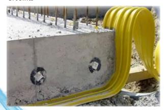
Expansion joints (if any) will be provided in the base slab/ and walls. Water stop of approved type and size will be provided above the blinding/formwork. Standard T, L etc. pieces, where required, will be used for joining the water stop.
