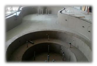
The surface shall be saturated with water and any standing water shall be removed. A thin layer of cement slurry shall be applied to the surface. Floating and wooden trowelling shall begin when the water sheen has disappeared, and when the mix has stiffened sufficiently to prevent excess fine material from working to the surface.
