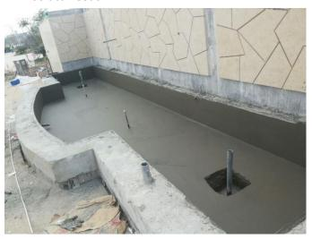
The surface shall be saturated with water and any standing water shall be removed. A thin layer of cement slurry shall be applied to the surface. Floating and wooden trowelling shall begin when the water sheen has disappeared, and when the mix has stiffened sufficiently to prevent excess fine material from working to the surface.
