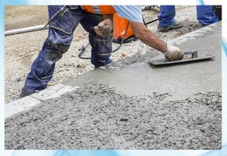
An approved mix design shall be used for affecting these works. Joints will be left at approx. 45 deg. angle and scarified with a sharp toothed trowel to ensure proper bonding at the joints. Any rebound / loose material will be completely cleaned and removed. After the concrete has begun to harden it should be protected from quick drying with hessian sheeting and wetted continuously. Curing of the concrete will be continued for a minimum of 7 days from the time of casting.
