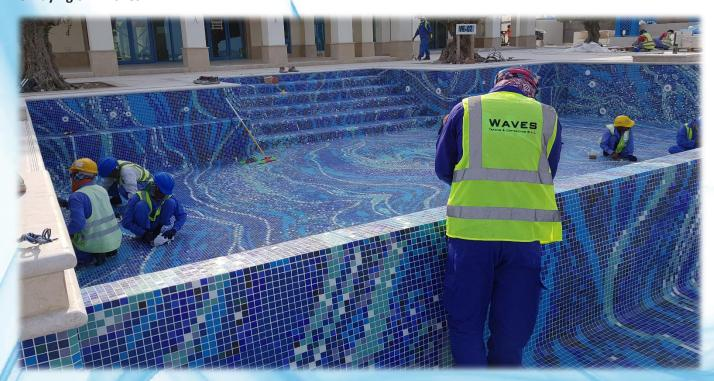
Work should be planned to start fixing at the top of the areas to be covered. The precise recommendations of the adhesive manufacturer should be followed concerning the suitability of the background, the mixing procedure, the method of use, the thickness of adhesive and the open time after spreading. It is important to the appearance of the finished that unsightly cut are avoided and that joints are of a uniform width.
