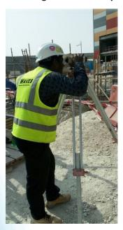
A setting out survey involves the marking out of any physical feature that appears on an engineering plan, in its correct position on the ground. These surveys are normally required during the construction of Water Features
