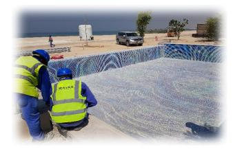
The coping will be bedded on a site mixed mortar of cement, washed aggregate and mixed with water as required installed approximately 25mm thick as a levelling course. A thin bed of the tile adhesive is installed on the mortar bed while it is still green and the coping/edging is set over this to line and level. All joints in the coping will be grouted.
