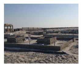
Form work for the outer edge of the base slab and walls will be in the form of hollow blocks laid on cement sand mortar on the blinding concrete. The constructed block work will be left as sacrificial formwork. Areas where both sides of the wall are exposed and / or are restricted, conventional formwork with timber will be used or expamet 'HIRIB' will be tied to the rebar as a permanent in-situ formwork.
