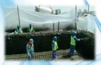
An approved mix design shall be used for affecting these works. Joints will be left at approx. 45 deg. angle and scarified with a sharp toothed trowel to ensure proper bonding at the joints. Any rebound / loose material will be completely cleaned and removed. After the concrete has begun to harden it should be protected from quick drying with hessian sheeting and wetted continuously. Curing of the concrete will be continued for a minimum of 7 days from the time of casting.
