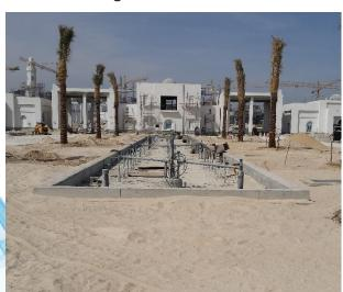
After the completion of the compaction and testing of the final layer, trenches for laying all the UPVC pipework below the base slab will be excavated and formwork in sacrificial block work constructed for the sumps. All pipework will be laid as per approved drawings and supplier's specifications, pressure tested for a minimum period of 24 hours prior to backfilling and levelling to the required profile.
