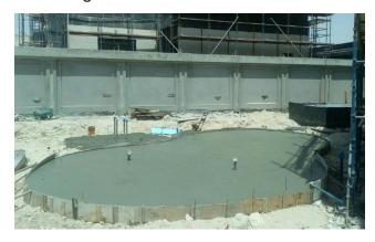
Blinding concrete to the required thickness as approved will be laid on a layer of 1000g polythene sheet over the prepared surface. The blinding concrete will extend a minimum of 200mm beyond the edge of the base slab. This is for the installation of sacrificial block work.
