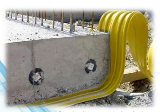
Expansion joints (if any) will be provided in the base slab/ and walls. Waterstop of approved type and size will be provided above the blinding/formwork. Standard T, L etc. pieces, where required, will be used for joining the waterstop.
