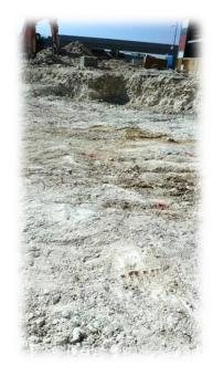
Soon after the survey, cleaning and clearing the existing grade will start. All contaminated and waste materials will be removed and disposed ofsite. Before filling (if required) commences, the sub- grade will be levelled, watered, compacted and tested.
