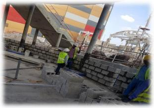
Formwork for the outer edge of the base slab and walls will be in the form of hollow blocks laid on cement sand mortar on the blinding concrete. The constructed block work will be left as sacrificial formwork. Areas where both sides of the wall are exposed and / or are restricted, conventional formwork with timber will be used or expamet 'HIRIB' will be tied to the rebar as a permanent insitu formwork.
