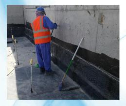
For horizontal & vertical waterproofing membrane application, a single layer of modified bituminous membrane shall be laid fully torched on blinding concrete & hollow block respectively. Waterproofing membrane will be protected by concrete screed for horizontal surfaces and protection board for vertical surfaces. Both waterproofing membrane and protection board will be installed by using cylinder fed propane gas torch.
