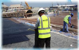
For horizontal & vertical waterproofing membrane application, a single layer of modified bituminous membrane shall be laid fully torched on blinding concrete & hollow block respectively. Waterproofing membrane will be protected by concrete screed for horizontal surfaces and protection board for vertical surfaces. Both waterproofing membrane and protection board will be installed by using cylinder fed propane gas torch.
