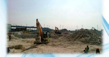
The area to be excavated shall be properly marked and clear before starting the works. As soon as the excavation reaches the required depth/elevation the surface shall be leveled and shall be compacted to required density. Before the compaction starts, it shall make sure that the excavated level is free from standing water or excessive moisture content.
