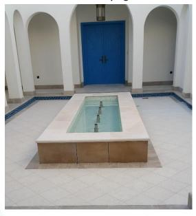
The coping will be bedded on a site mixed mortar of cement, washed aggregate and mixed with water as required installed approximately 25mm thick as a levelling course. A thin bed of the tile adhesive is installed on the mortar bed while it is still green and the coping/edging is set over this to line and level. All joints in the coping will be grouted.
