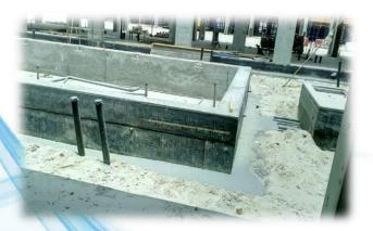
After curing of the concrete, cleaning and clearing the surrounds will start. All contaminated and waste materials will be removed and disposed of-site. Before back- filling commences, the subgrade will be watered, levelled and compacted.
