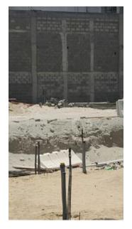
Soon after the survey, cleaning and clearing the existing grade will start. All contaminated and waste materials will be removed and disposed ofsite. Before filling (if required) commences, the sub- grade will be watered, levelled. compacted and tested.
