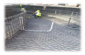
All rebar will be cut, bent and stored according to the relevant code of practice. All rebar will be placed to the required spacing as per design and tied with binding wire. Cover blocks will be used to obtain the required cover to the rebar. Two layers of rebar will be separated with 'chairs' made of 8/10mm rebar. Lapp lengths of 50 times the diameter of the bar will be provided.
